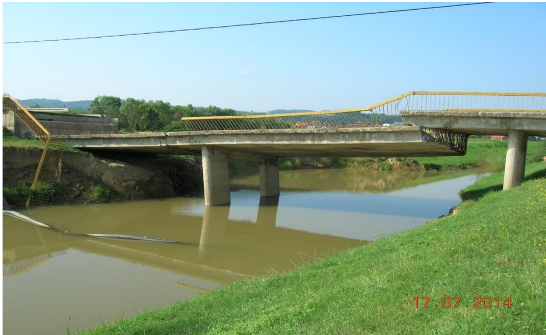
Photo 1. Old bridge (View from the downstream side)
