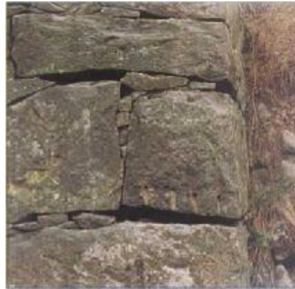
Fig. Loss of snecks.
