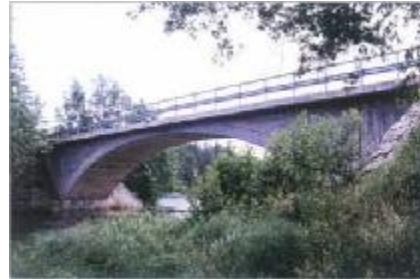
Fig. Concrete arch bridge
