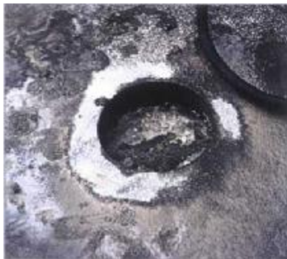
Fig. Core drilled window.
