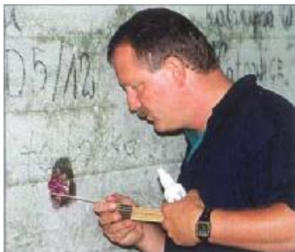
Fig. Measurement of depth of carbonation.
