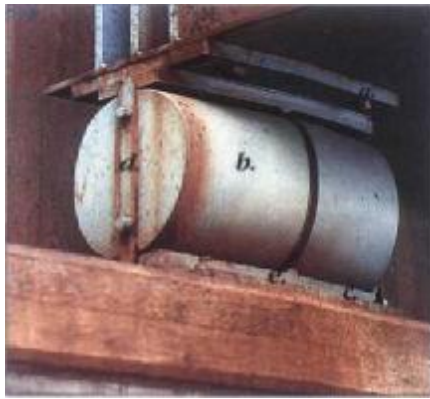
Fig. a. Upper bearing plate b. Roller c. Lower bearing plate d. Guide bar e. Locating bar
