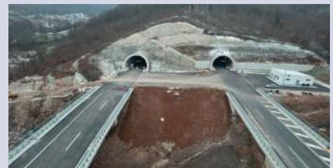
cross from one tunnel tube to the other in the event of an emergency, which can also be used by emergency vehicles. Each tunnel tube has two emergency niches, extensions for removing broken down vehicles.
