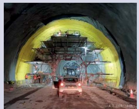
Tunnel works are carried out in complex geological conditions, using a construction technology called the "New Austrian Method" (NATM), which involves mapping the tunnel excavation and measuring deformations according to the principle of 3 examples.
