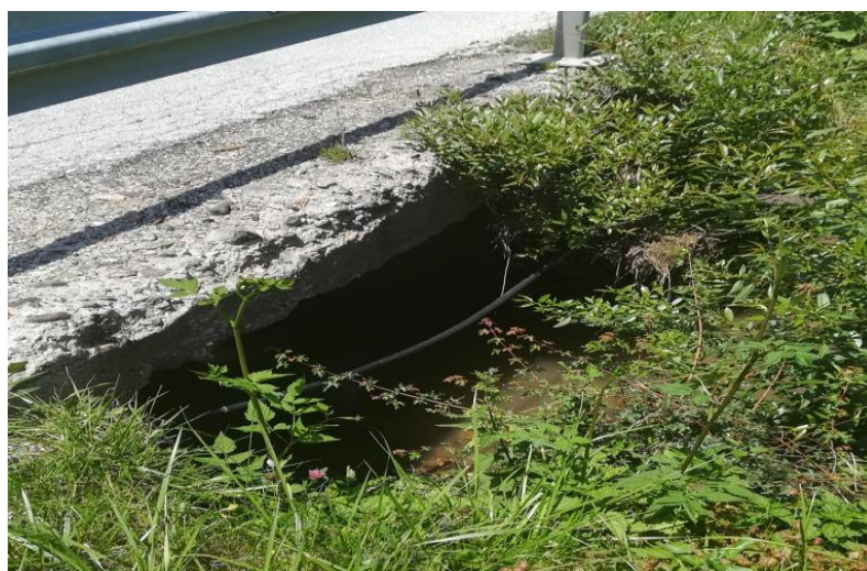
Picture 11. Box culvert on km 90+205.79 (Osaonicki stream)
