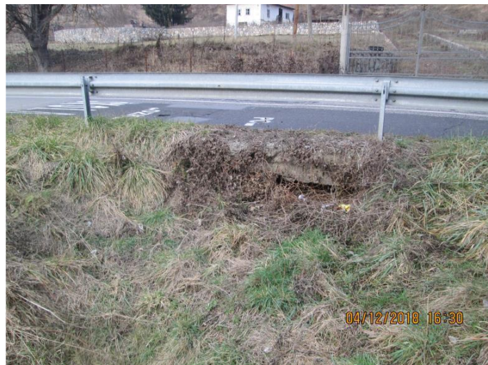
Picture 10. Box culvert on km 88+539.30
