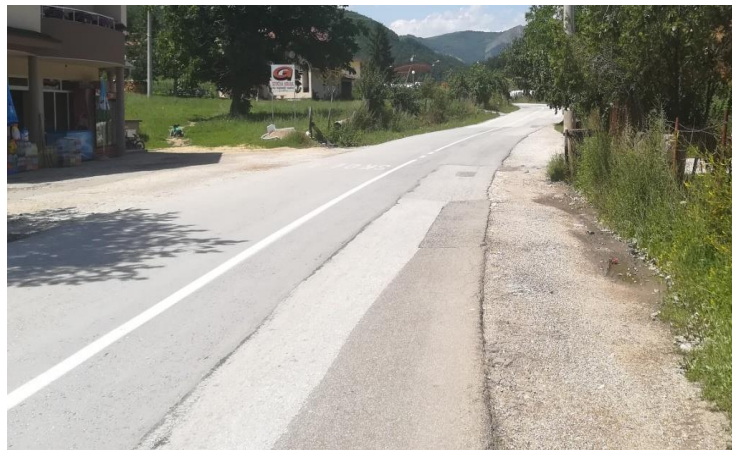
Picture 16. Roadway detail in the settlement of Bele Vode
