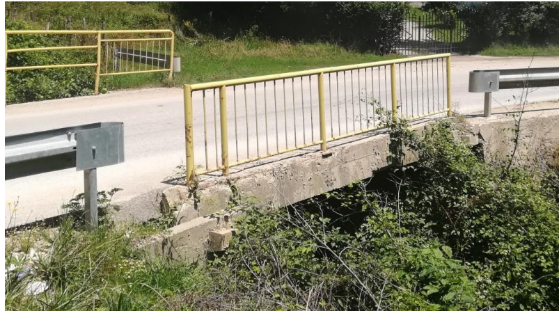
Picture 12. Box culvert on km 99+046- Kukavicka River
