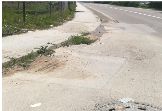
Picture 22. Existing "closed" drainage system
