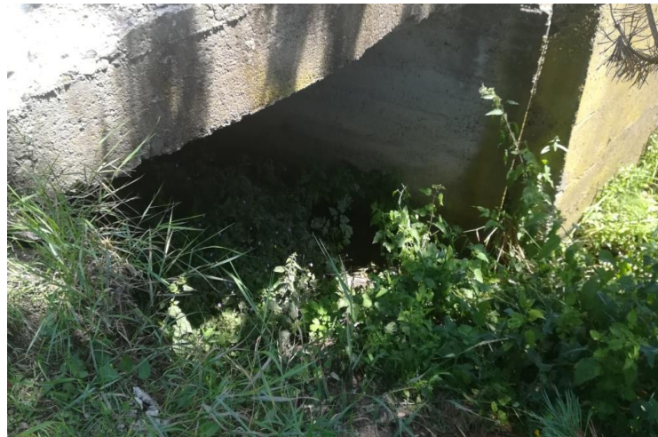
Picture 7. Box culvert on km 84+487.20 (Belovodski stream)
