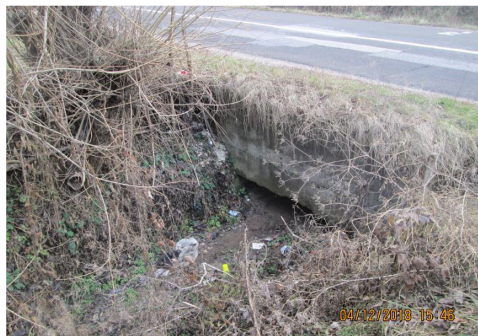
Picture 8. Box culvert on km 85+878.88 (Cebinski stream)
