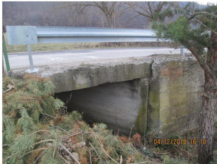
Picture 9. Box culvert on km 87+317.02 (Bezimeni stream Janca)
