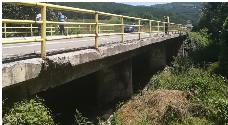
Picture 6. Bridge over the Ljucka River km 86+265
