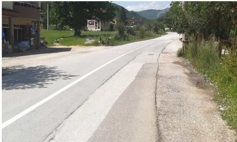
Picture 29. Detail of the road in the settlement Bele Vode
