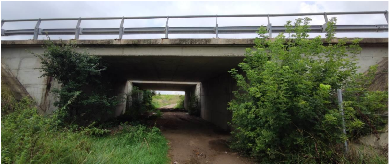
Picture 31- Side view to the bridge, of the local road
