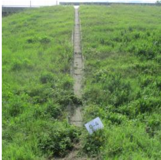
Picture 25 - Typical appearance of the grip condition
