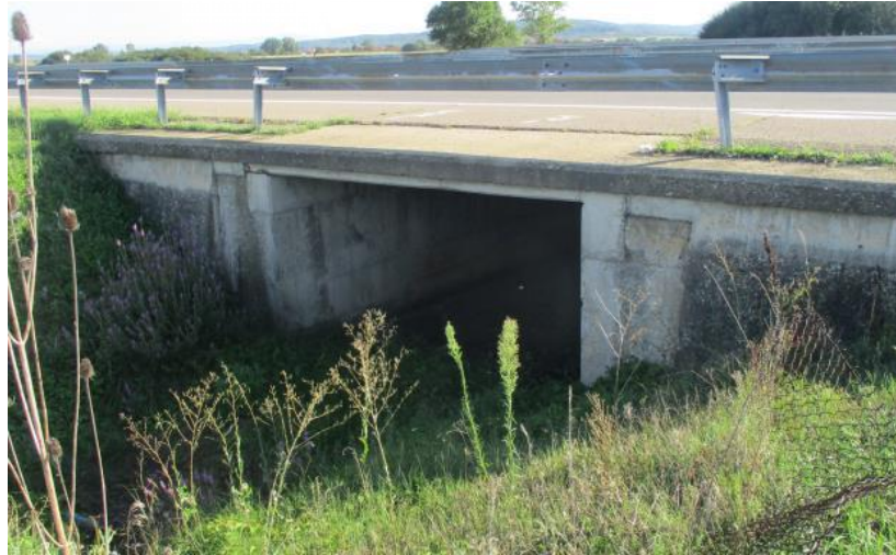
Picture 10 - Box culvert at the station km 454+935
