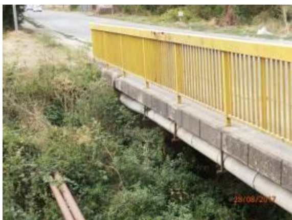
Figure 3.13 - Bridge over the Krajkovacka River
