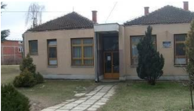
Figure 3.2 - Primary school "Jastrebacki partizani" in Merosina
