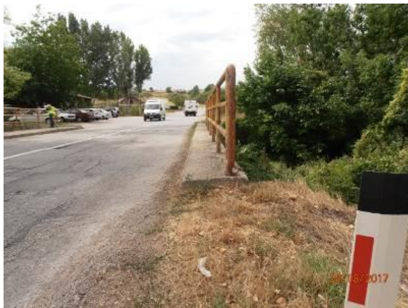
Figure 1.6 – bridge over the Jugbogdanovacka River
