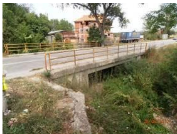
Figure 3.14 - Bridge over the Jugbogdanovacka River
