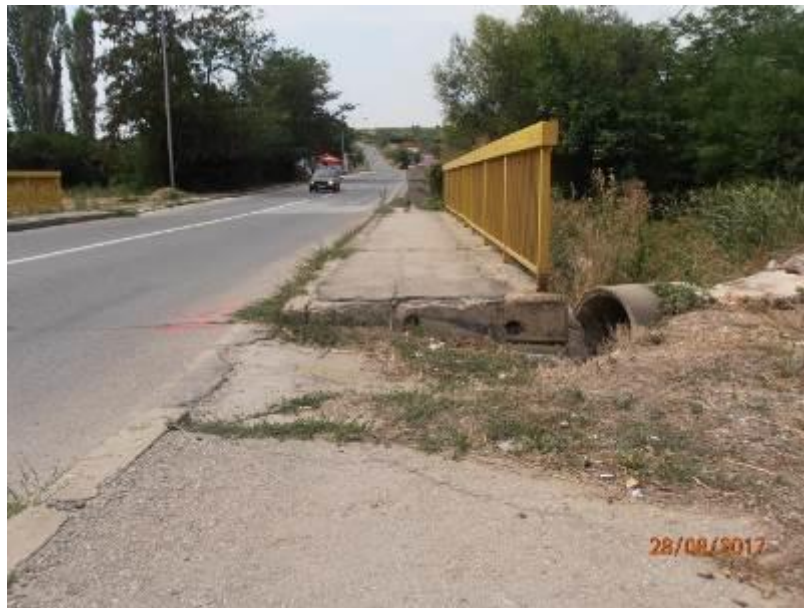
Figure 1.5 – bridge over the Krajkovacka River
