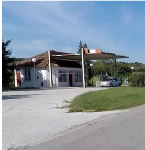
Figure 2-11 Gas station in Misljenovac, at km 53+185
