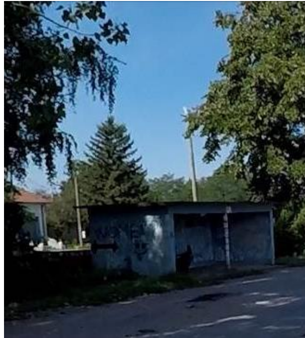
Figure 2-7 Bus stop, Misljenovac, at km 53+485
