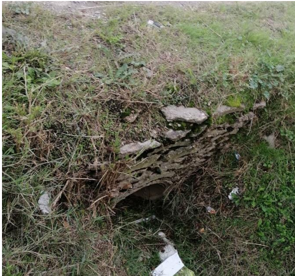
Figure 2-34 Vaulted culvert, km 43+942
