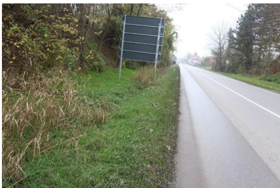
Figure 2-35 km ~20+000 the ditch covered in vegetation
