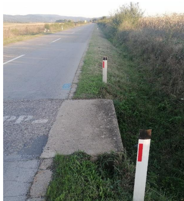
Figure 2-33 Box culvert and canal, km 48+495
