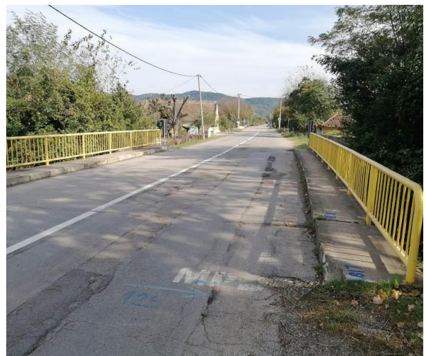
Figure 2-29 The bridge in Misljenovac
