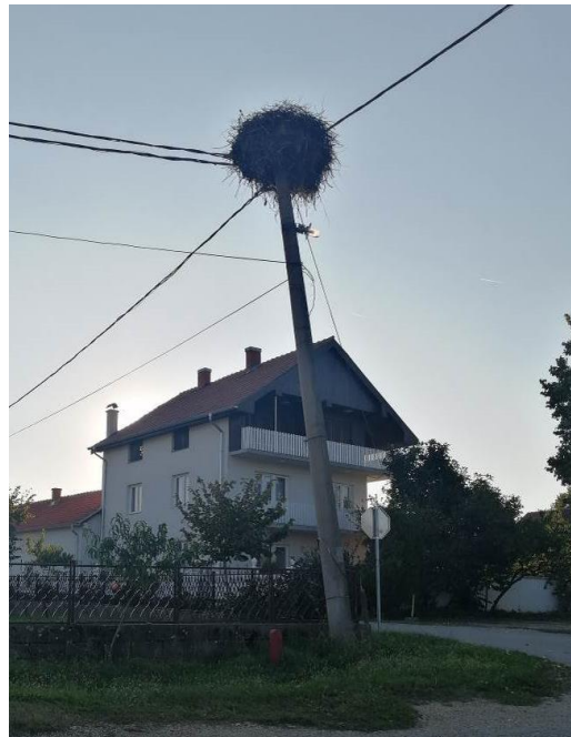
Figure 2-21 Mustapic, a stork nest on a public lighting pole, at km 50+970
