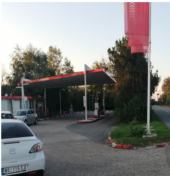
Figure 2-12 Gas station "Lukoil", Rabrovo, at km 47+890
