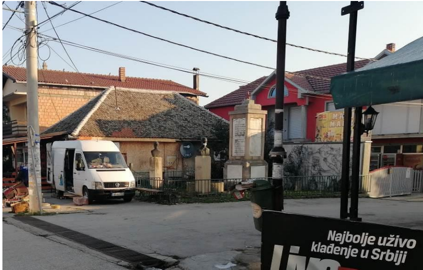
Figure 2-16 The monument to the fighters in the Second WW, in Rabrovo, at km 47+263
