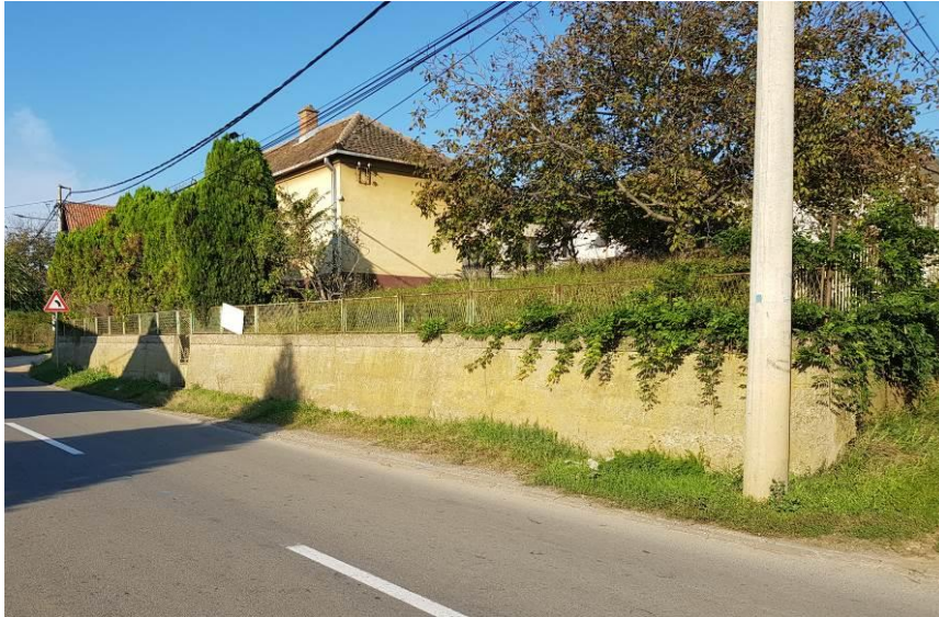
Figure 2-2 Retaining wall No 3, Rabrovo
