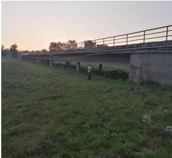
Figure 2-26 The bridge over the Mlava river
