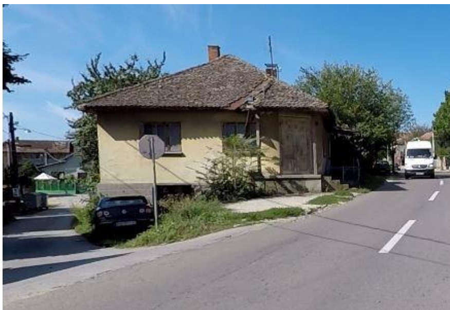
Figure 2-17 The house in Rabrovo where Serbian actress Zanka Stokic lived, at km 47+090
