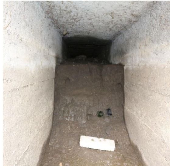
Figure 2-35 Culvert filled with material, km 31+151
