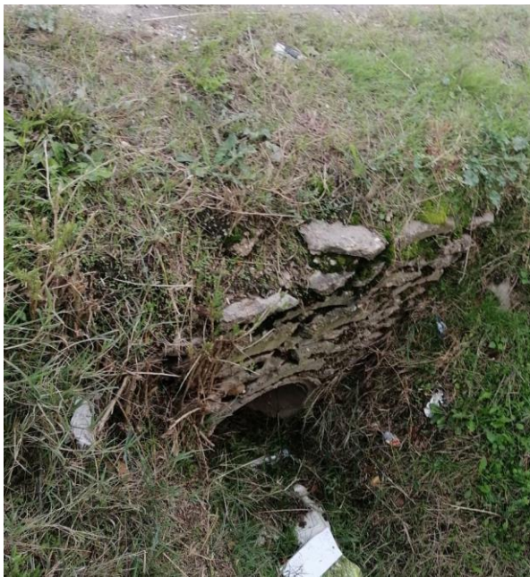
Figure 2-32 Pipe culvert, km 42+431
