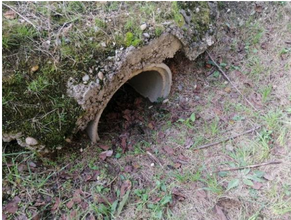
Figure 2-35 Pipe culvert at km 36+392
