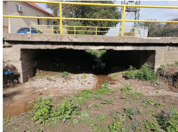
Figure 2-36 Box culvert, km 32+800
