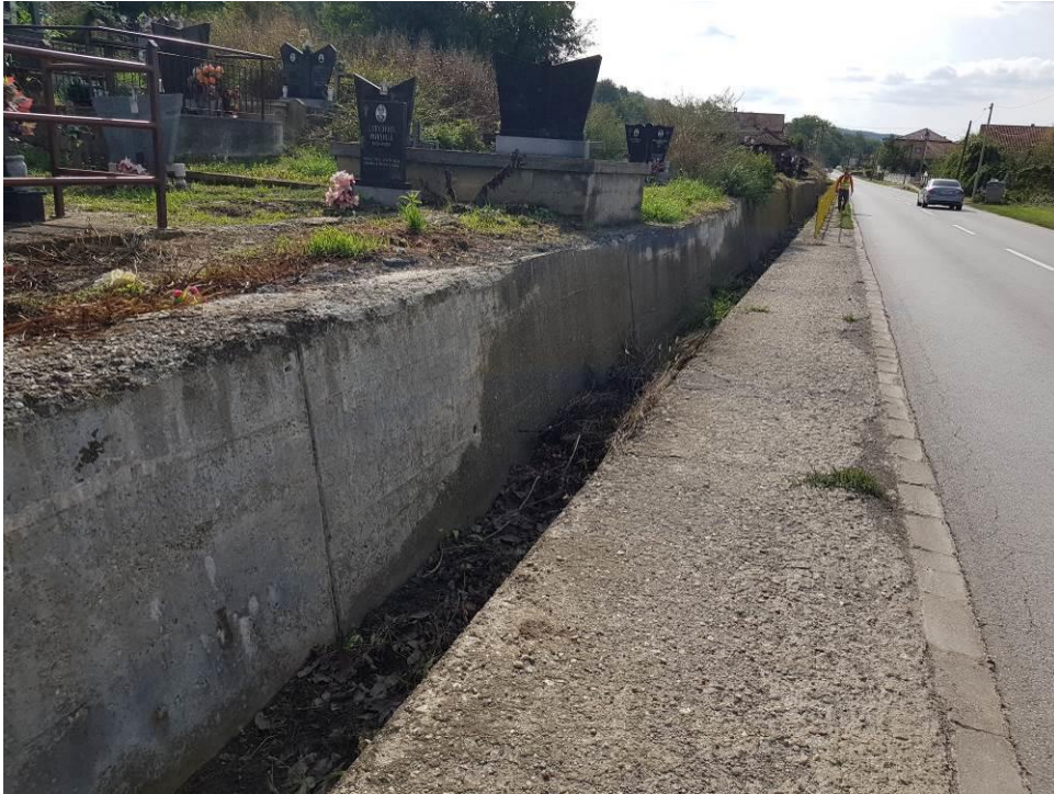
Figure 2-2 retaining wall No. 5, at Topolovnik graveyard
