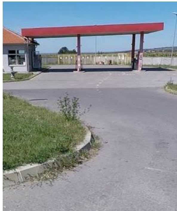
Figure 2-12 Gas station "MFK Petrol", at km 23+050
