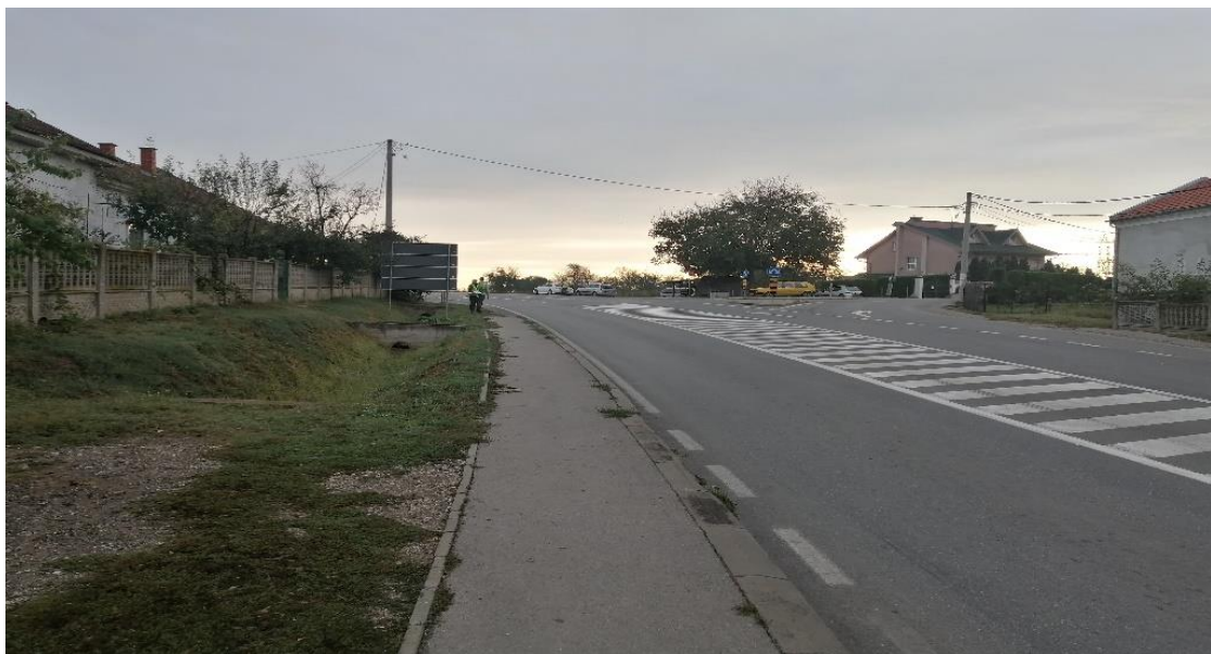
Figure 1-3 The beginning of the subject road section
