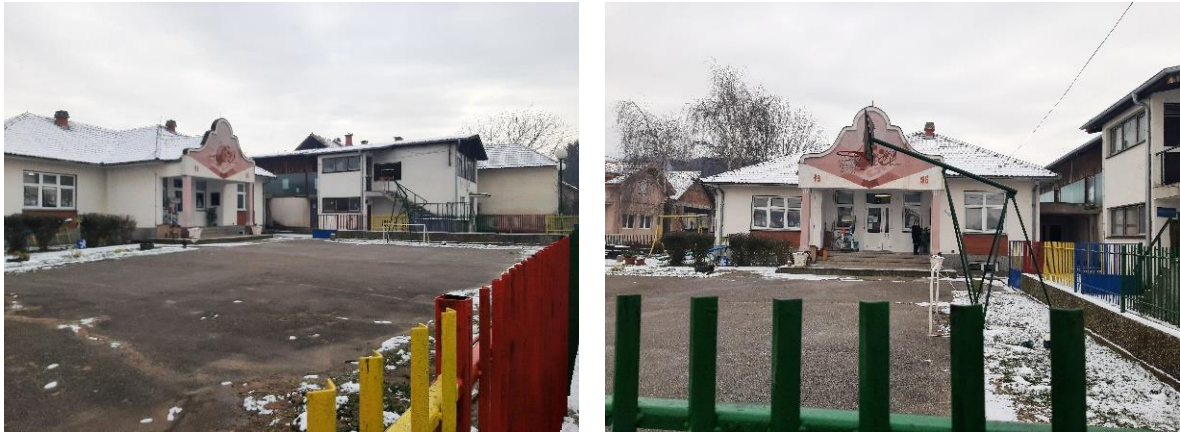
Figure 2-5 Elementary school Ivo Lola Ribar in Kumane, at km 34+835
