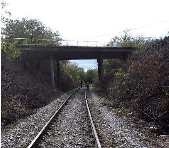
Figure 2-24 The overpass over the railway in Sirakovo settlement
