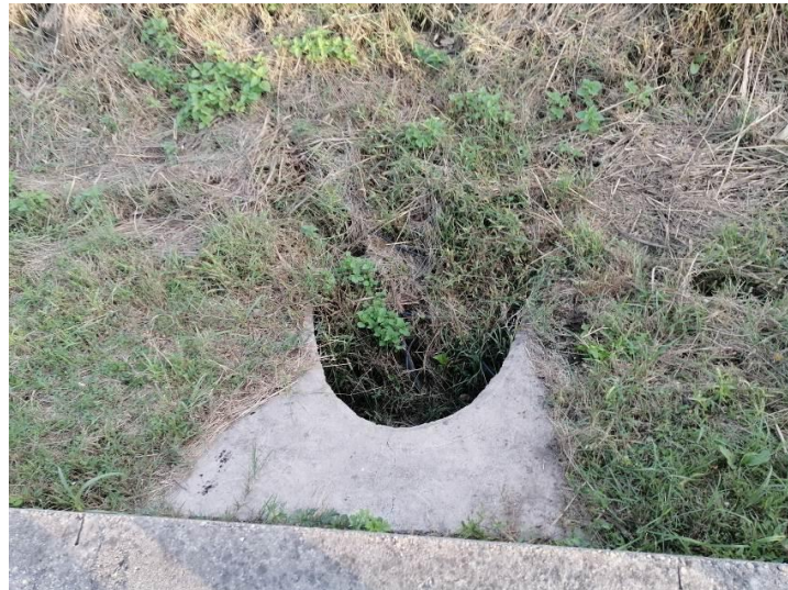
Figure 2-26 Arched culvert, at km 37+844
