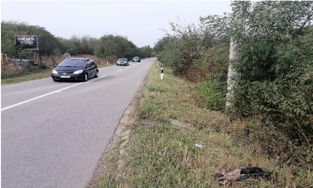
Figure 1-4 The end of the subject road section
