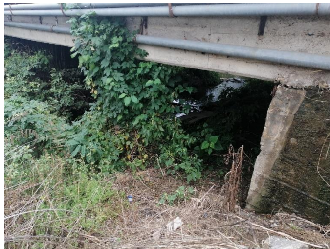
Figure 2-33 The bridge over the canal in Djurakovo settlement
