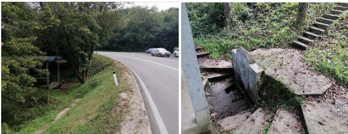
Figure 2-21 A fountain between Majilovac and Djurakovo, km 26+732
