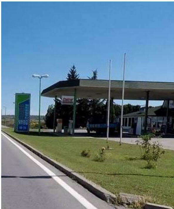
Figure 2-11 Gas station "Atlantik", at km 17+100
