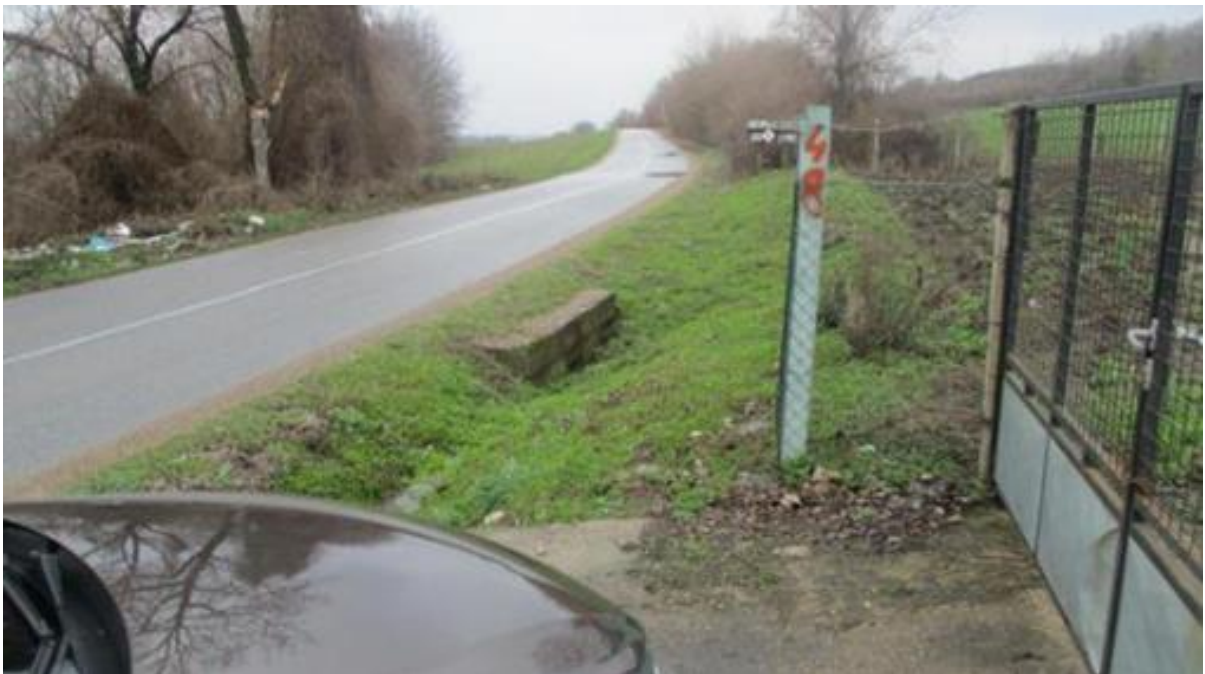
Figure 23. Waste dump - front of the culvert
