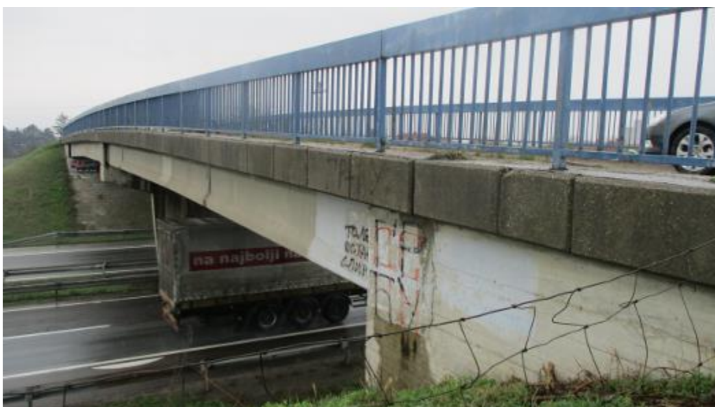
Figure 12. Overpass on the highway Beograd-Nis (Cuprija)
