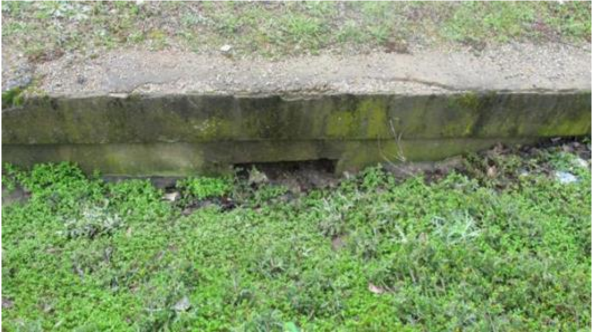
Figure 20. Burried culvert under the pavement
