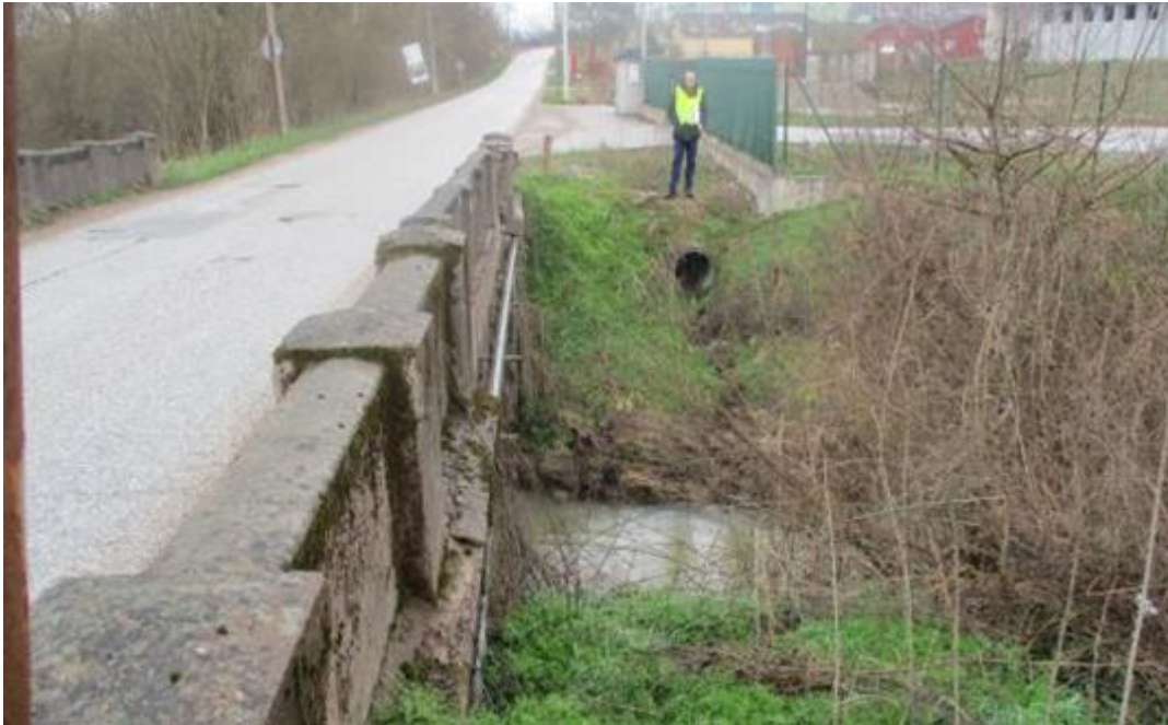
Figure 4. Concrete bridge over the river Dubnica
