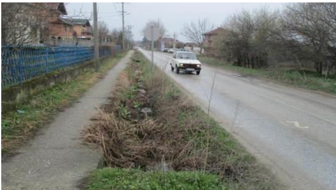
Figure 16. The existing roadway canal
