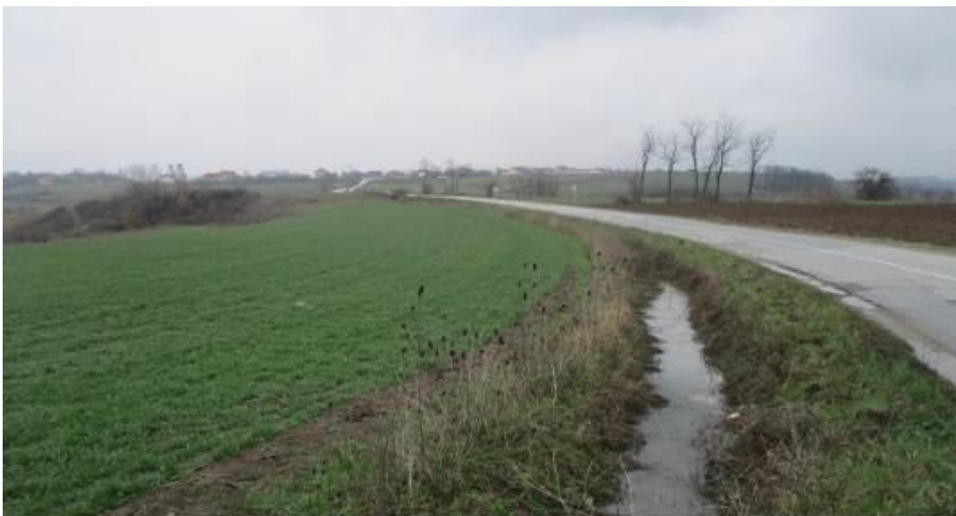
Figure 5. Existing road channels
