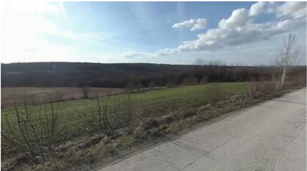
Figure 19. Drain down the slope of the embankment
