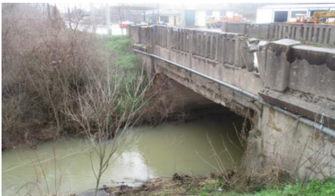
Figure 3. Concrete bridge over the river Dubnica
