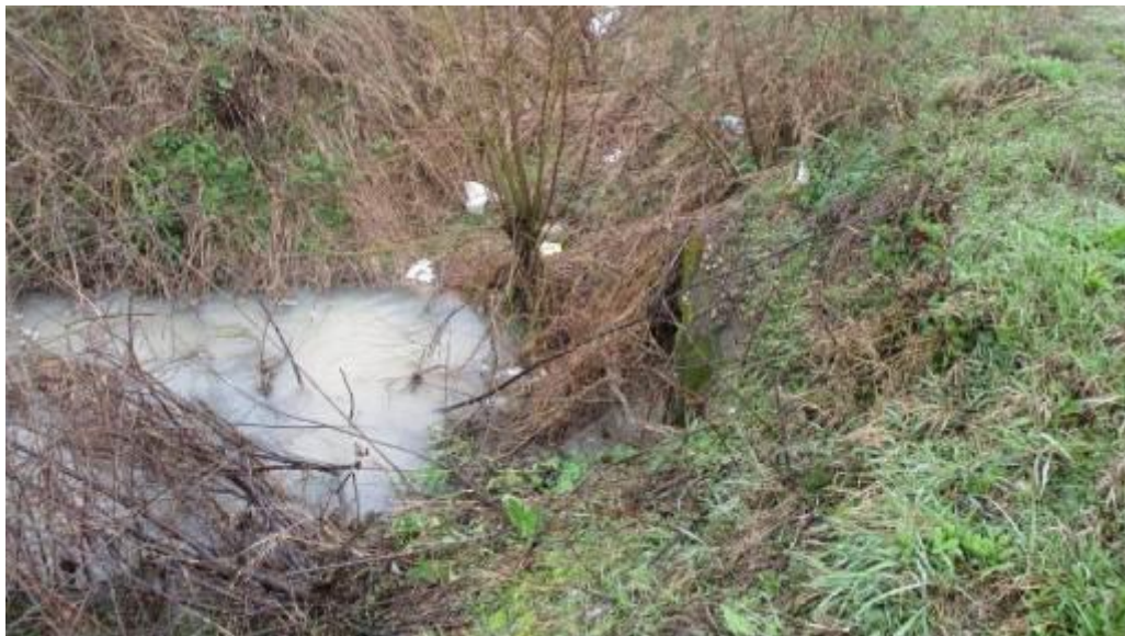
Figure 17. The existing culverts
