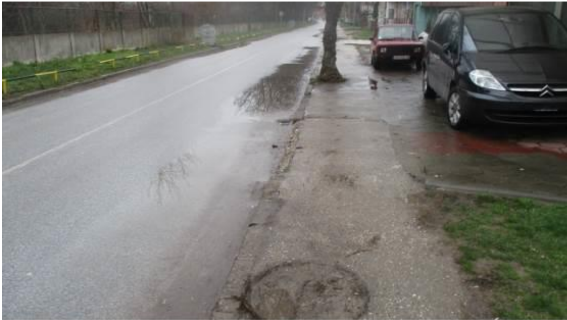
Figure 15. The existing roadway canal
