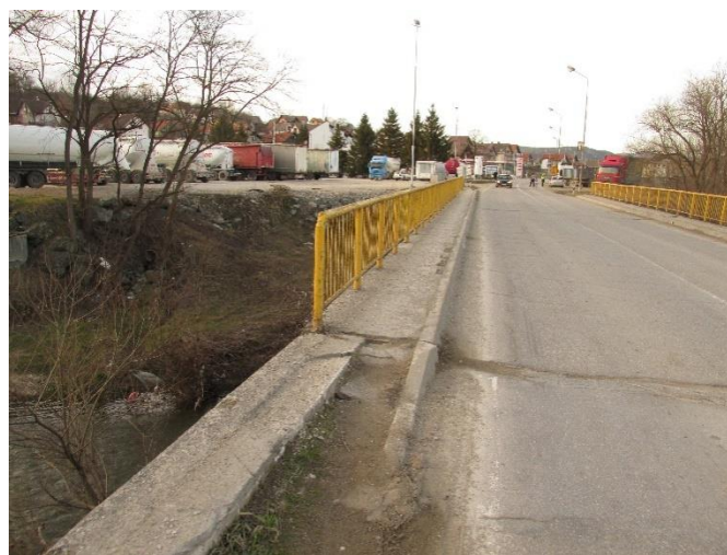
Figure 9. The Bridge over Kladoroba River in Kosjeric at ~ km 183+390
