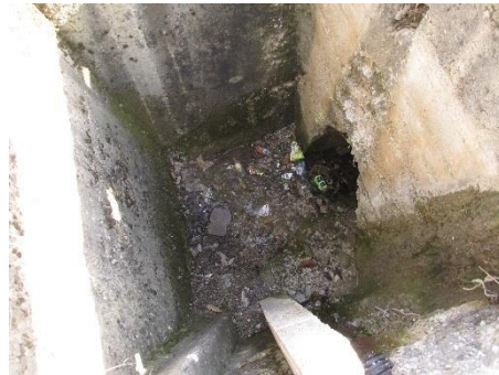
Figure 33. Combined culvert at ~ km 185+413
