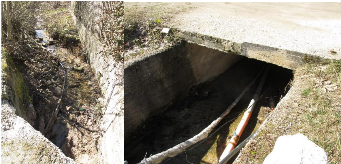
Figure 34. Slab culvert at ~ km 188+750
