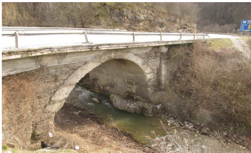
Figure 28. The Bridge over Gradnja creek near Kalenic at km 192+886
