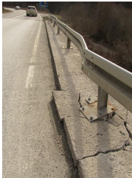
Figure 11. The Bridge over Gradnja creek near Kalenic at ~ km 192+886
