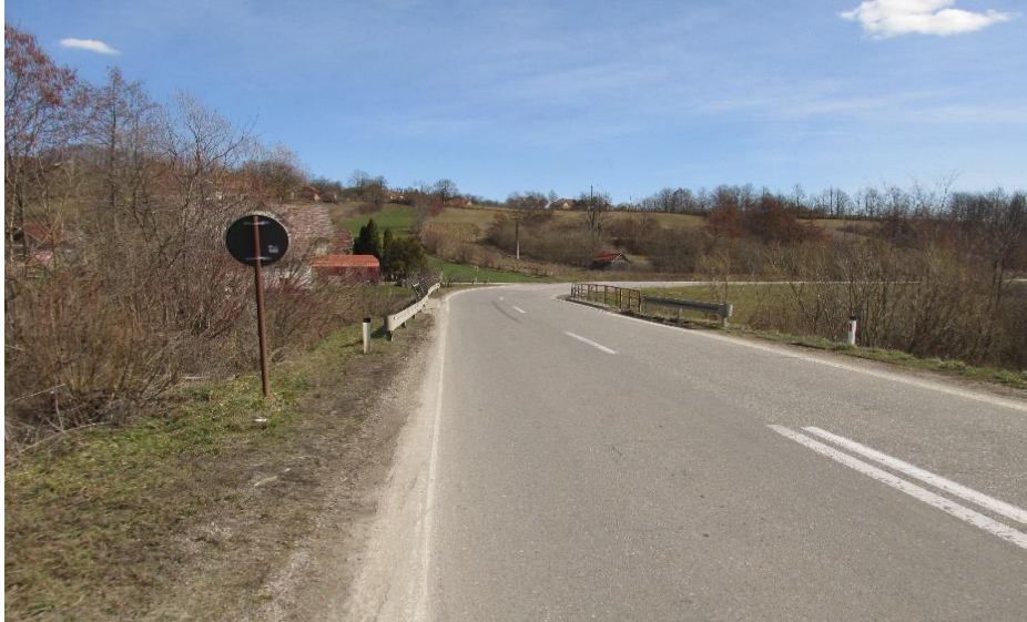
Figure 26. The Bridge over Nenadkovice River near Tubici at km 188+094
