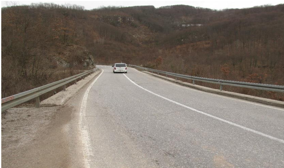
Figure 27. The Bridge over creek near Tubici at km 190+815
