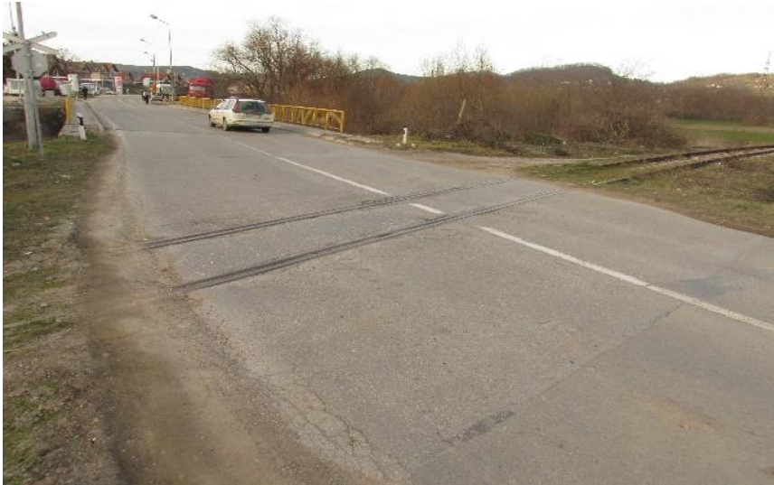
Figure 24. Railway spur track at ~ km 183+429
