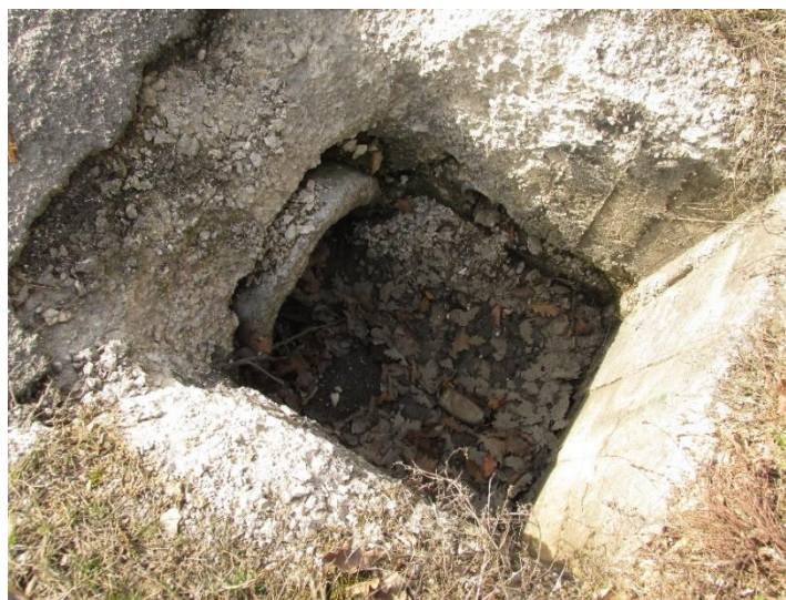
Figure 31. An example of inlet structure of the pipe culvert at ~ km 192+612
