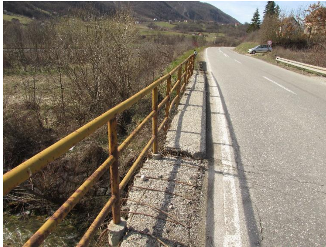
Figure 10. The Bridge over Nenadkovice River at ~ km 188+094
