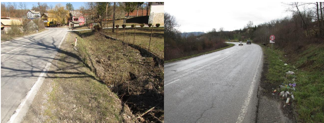
Figure 13. Canals on the observed road section
