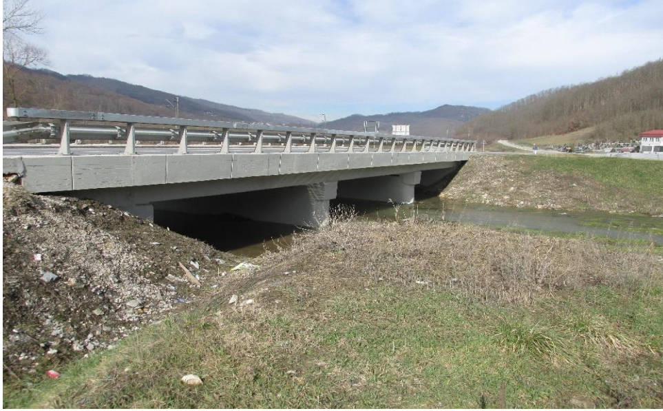
Figure 29. The Bridge over Dobrinjska River at km 198+247
