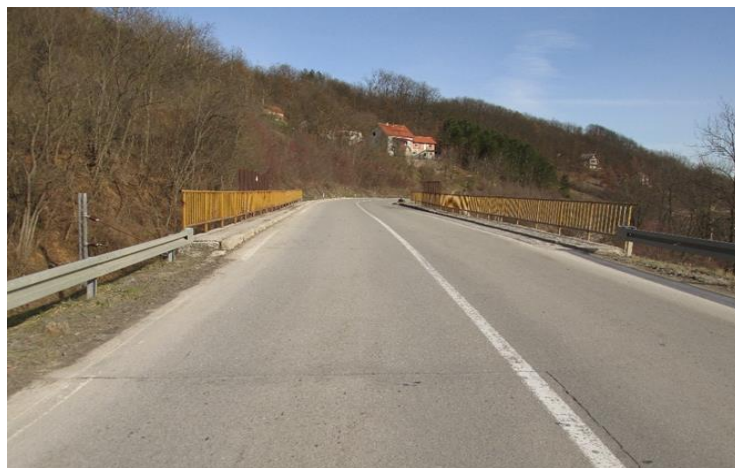
Figure 23. Overpass at Belgrade-Bar railway near Kosjeric
