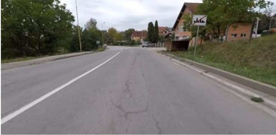
Figure 5. The end of the road section in Pozega
