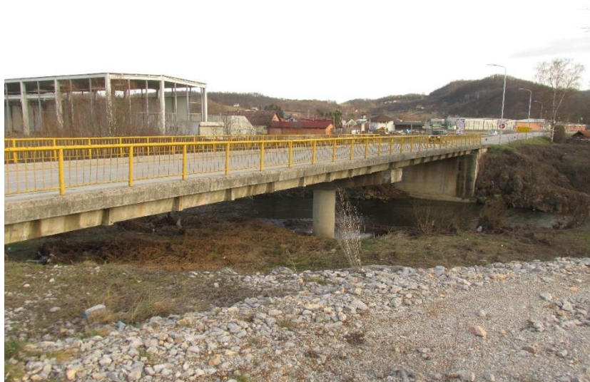
Figure 25. The Bridge over Kladoroba River in Kosjeric at km 183+390
