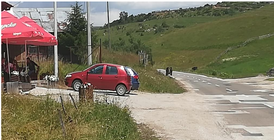
Picture 12. An example of damage to the subject section, the centre of Brnjica settlement
