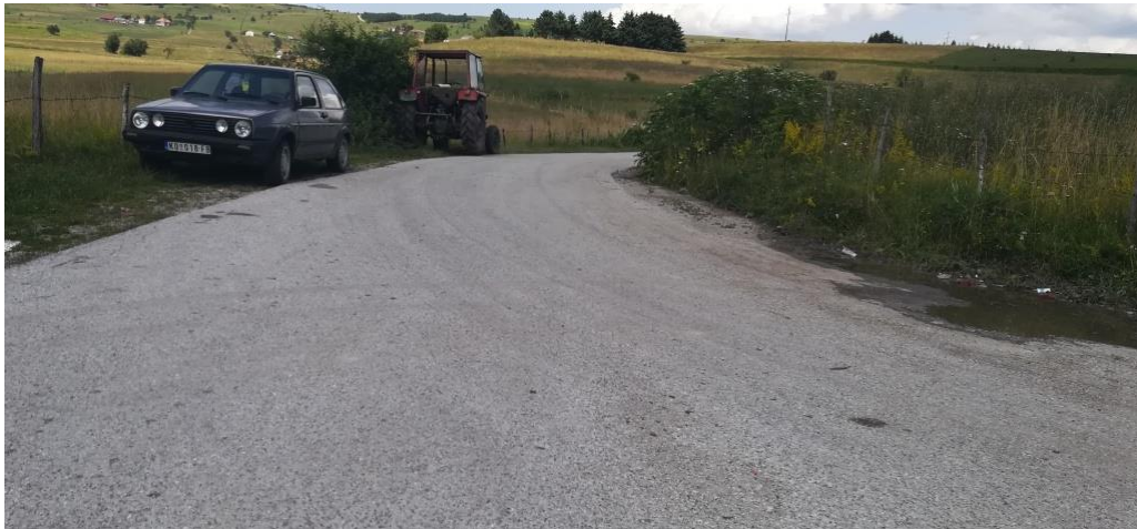
Picture 10. The local road for settlement Stup, km 67+440
