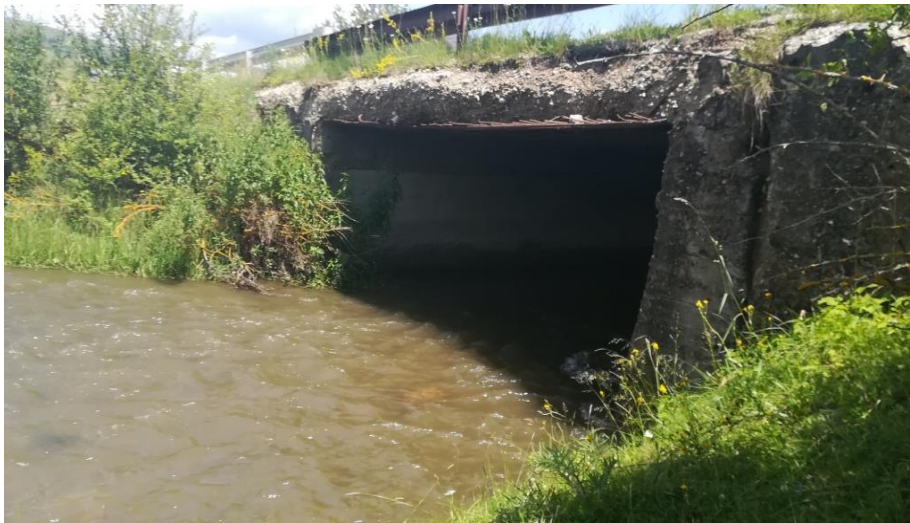
Picture 8. The bridge on the Brnjicka River, km 71+646
