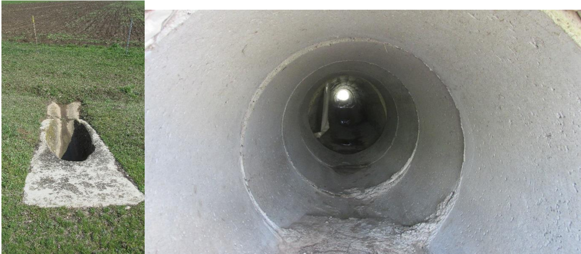
Figure 25. Pipe culvert at km 374+858
