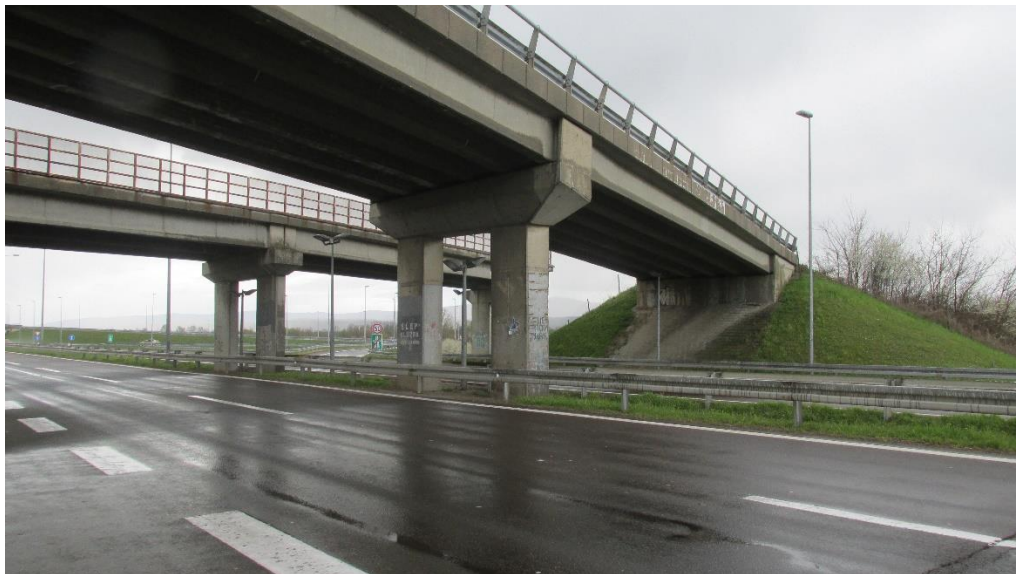
Figure 30. Overpass at km 405+110
