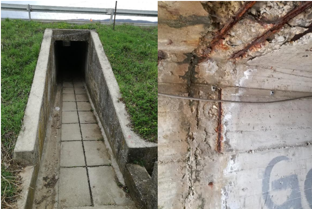
Figure 26. Slab pedestrian culvert at km 408+209
