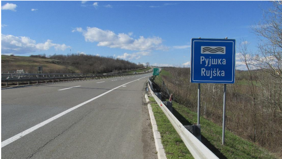
Figure 18. The Bridge over Rujška River at km 392+249
