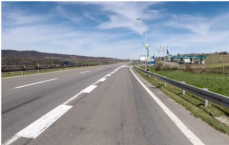
Figure 11. Petrol station "OMV" at km 390+100
