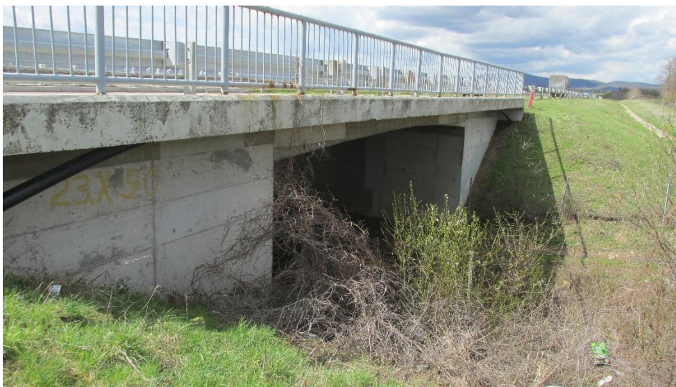
Figure 20. The Bridge over Suvi Creek at km 396+525
