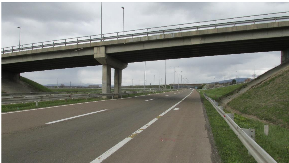
Figure 31. Overpass at km 405+460
