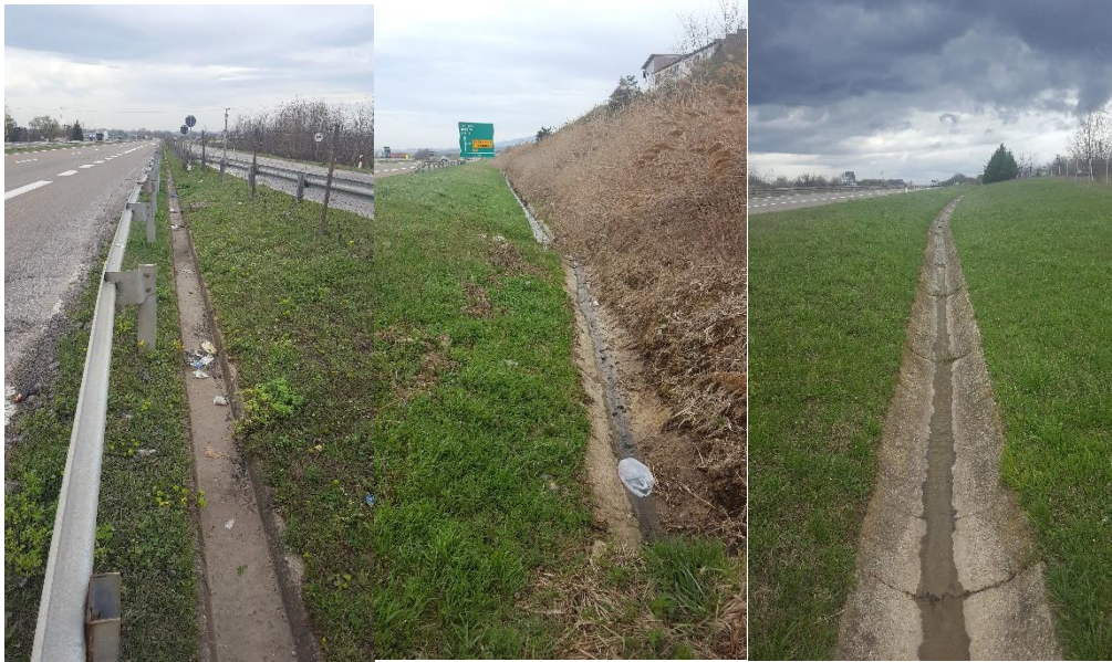
Figure 9. Concrete channels on the subject section
