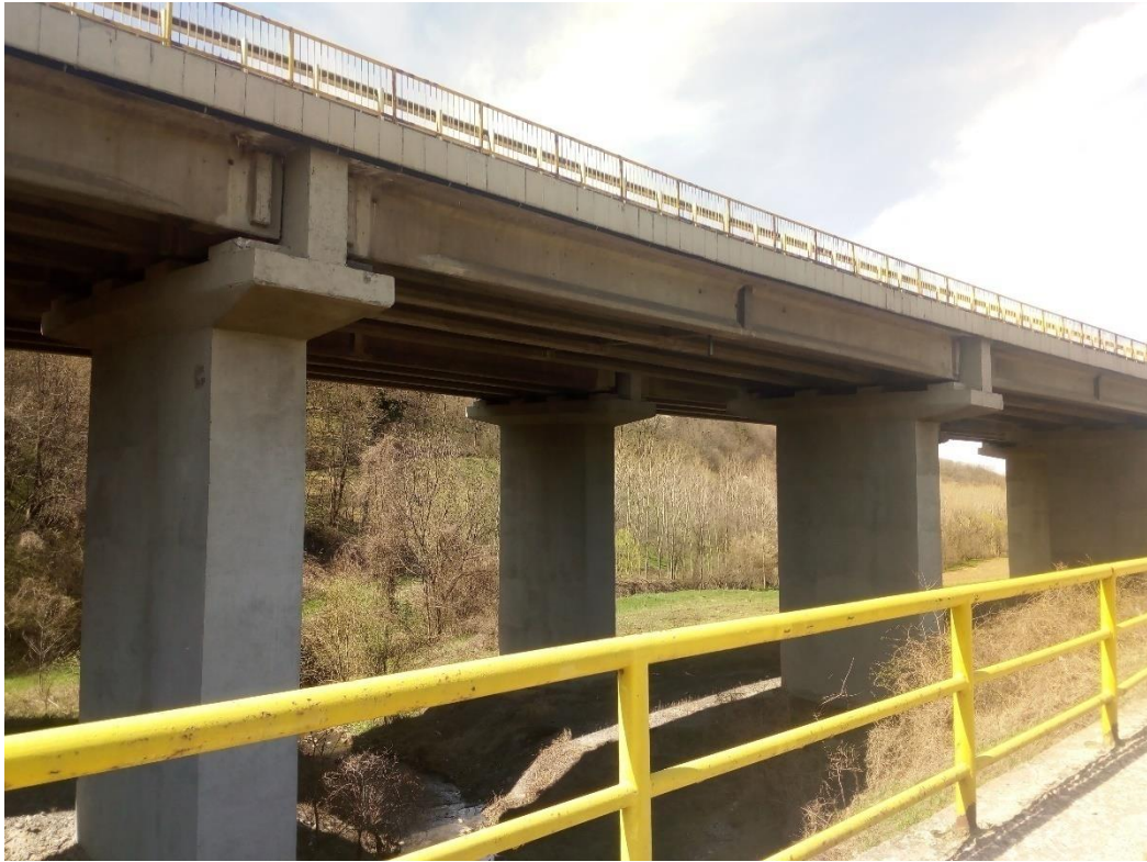
Figure 16. Ražanj Creek Viaduct at km 386+425
