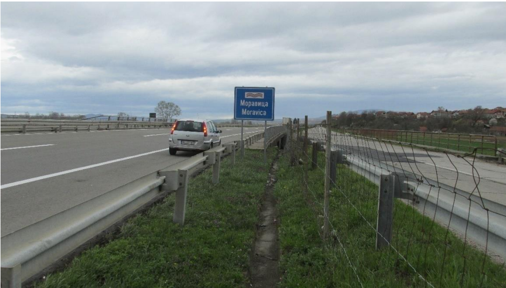
Figure 22. The Bridge over the Moravica River at km 407+758
