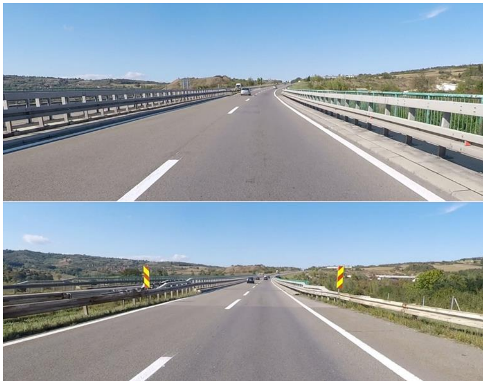
Figure 17. Ražanj Viaduct at km 388+163
