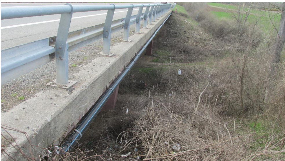
Figure 19. The Bridge over Drenovački Creek at km 394+029
