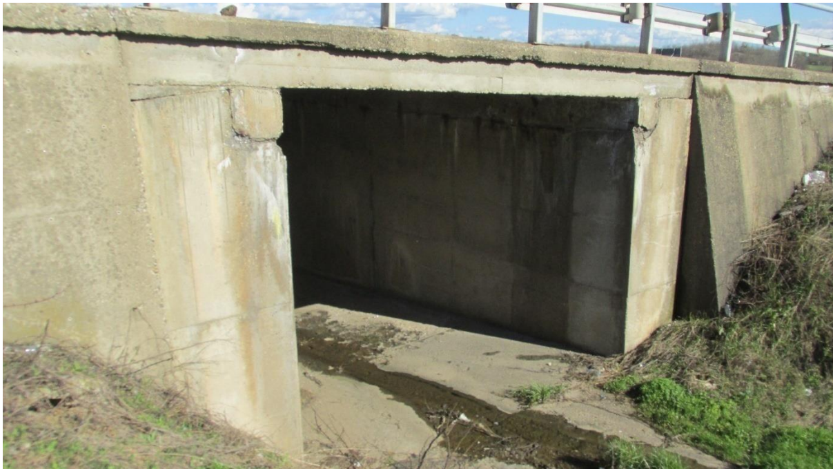
Figure 24. Slab culvert at km 391+622
