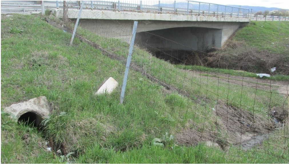
Figure 21. The Bridge over Rutevački Creek at km 398+480
