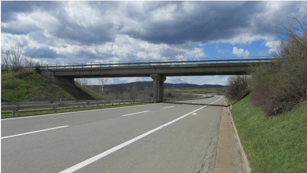
Figure 29. Overpass at km 394+182
