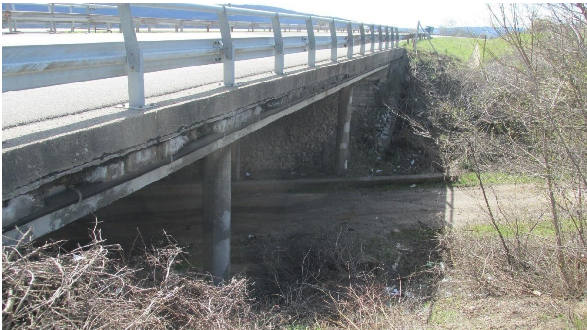
Figure 28. Overpass intersection Deligrad at km 393+248
