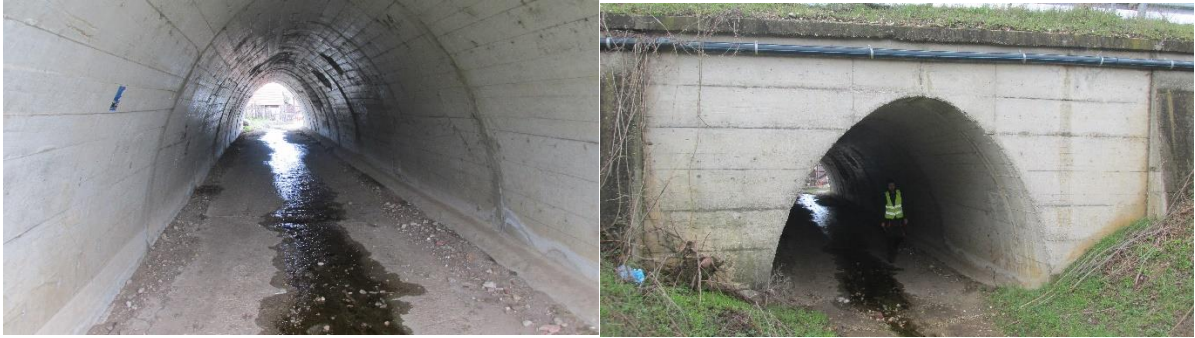
Figure 23. Arched culvert at km 402+203
