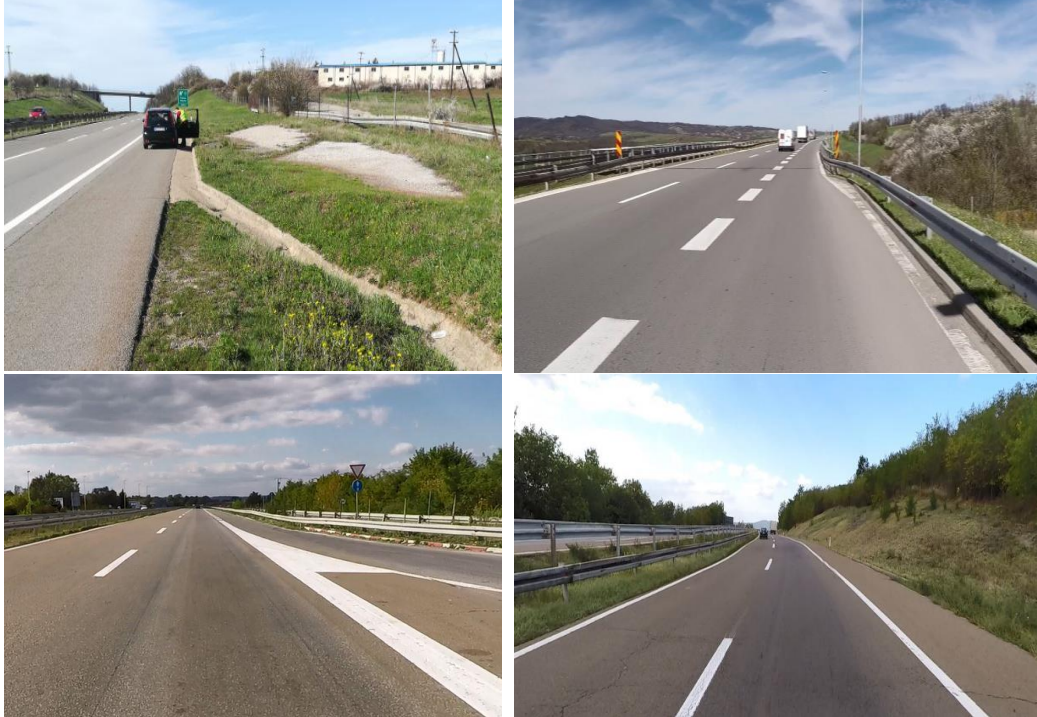
Figure 7. Typical parts of the subject section
