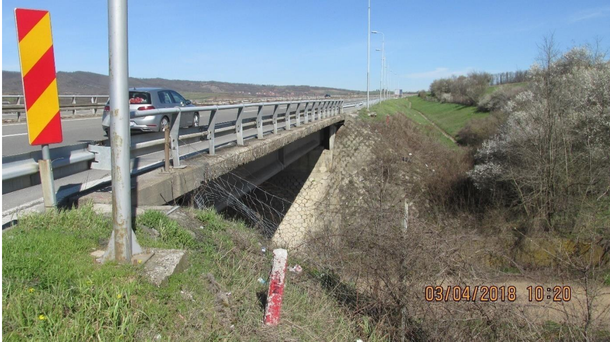
Figure 27. The bridge over the road Đunis – Ražanj at km 389+947
