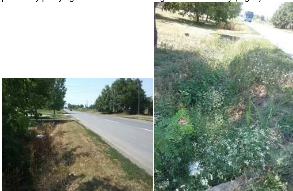
Figure 6 Self-absorbent ditches
