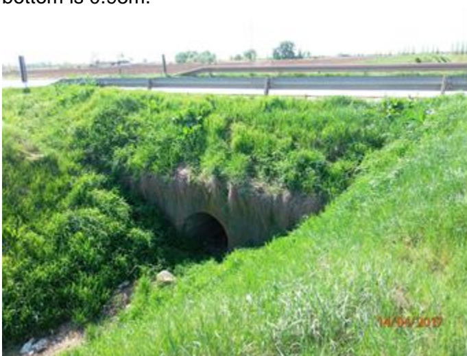
Figure 4 Intersection of the canal and road at the road chainage km 82+475
