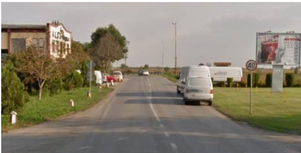
Figure 1. The beginning of the road section - exit from the municipality Vrbas
