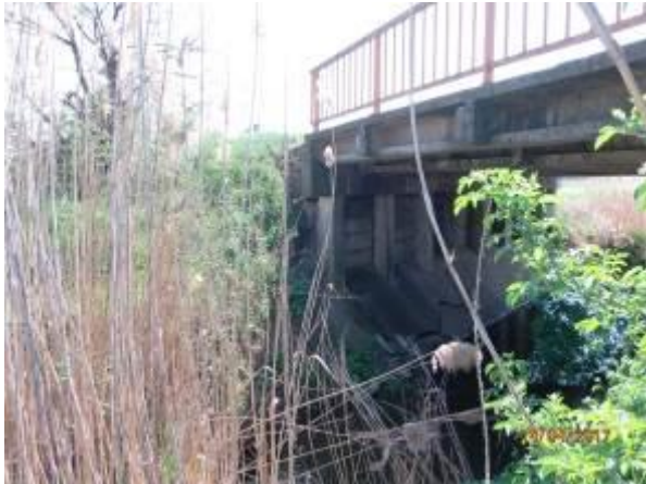
Figure 3 Bridge at the road chainage km 80+525
