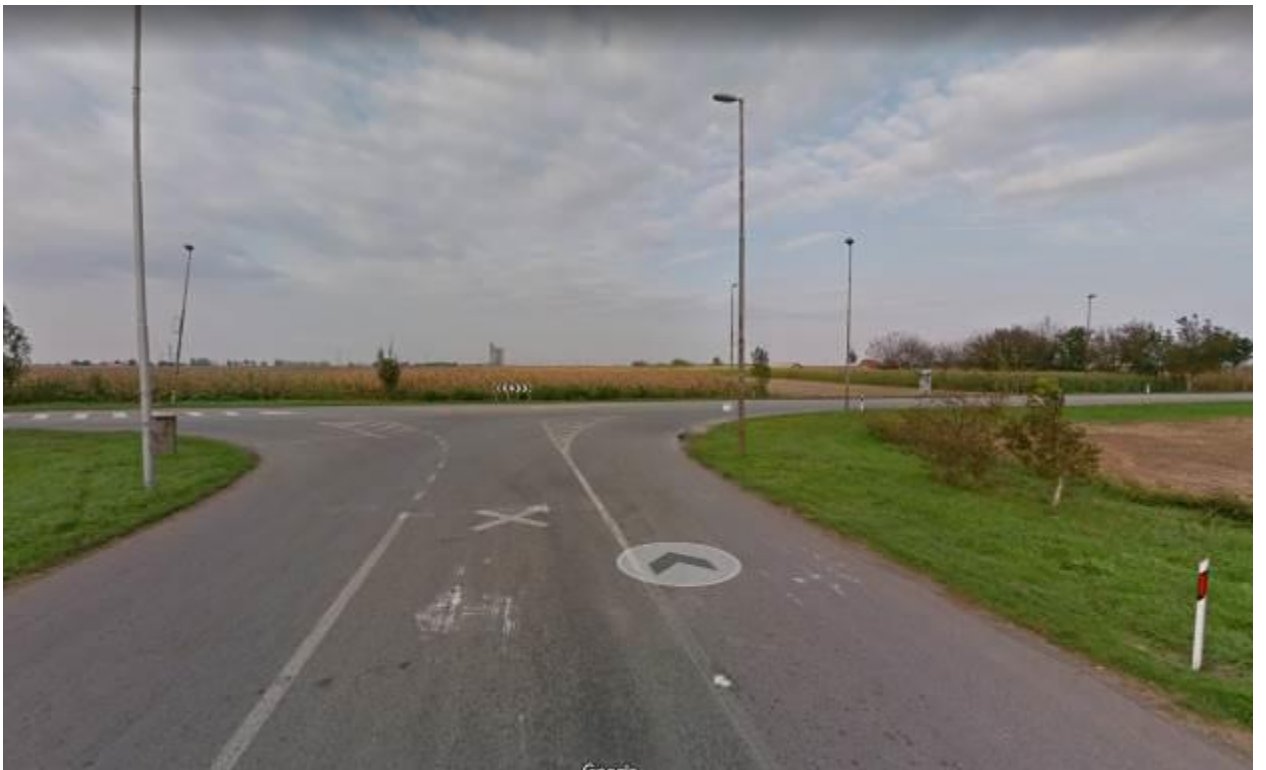
Figure 13 Three-way intersection at km 80+010
