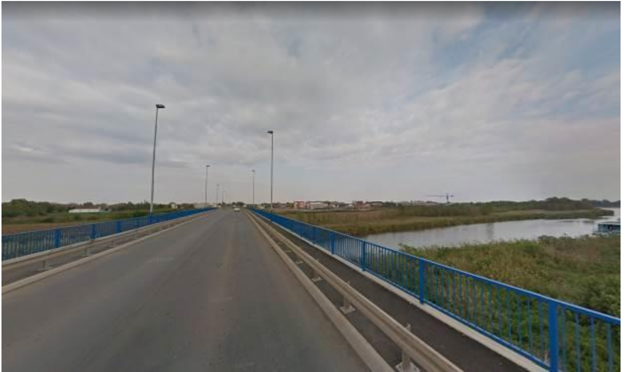
Figure 12 Bridge over Canal Veliki Backi
