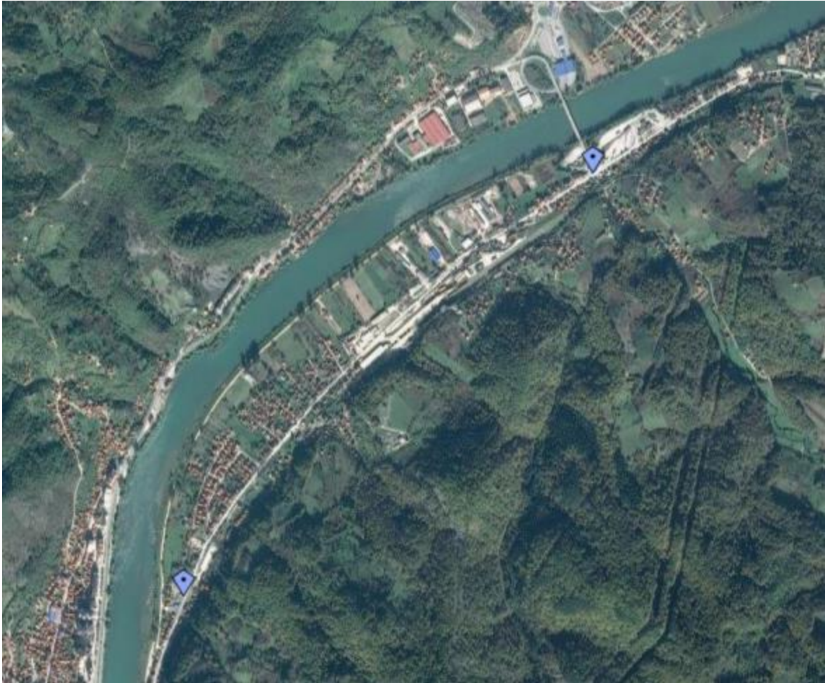
Picture 2. Ortho photo image sections of Mali Zvornik - Gracanica, from the border crossing "Karakaj" towards Mali Zvornik to 'NIS' petrol station, from km 0 + 000 to km 1 + 800, on the state road IB Class no. 28 Mali Zvornik – Uzice
