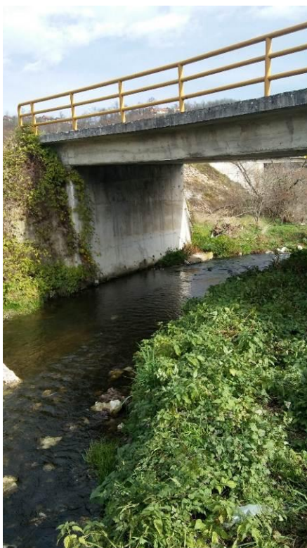
Figure 14: One of the bridges along the subject road section
