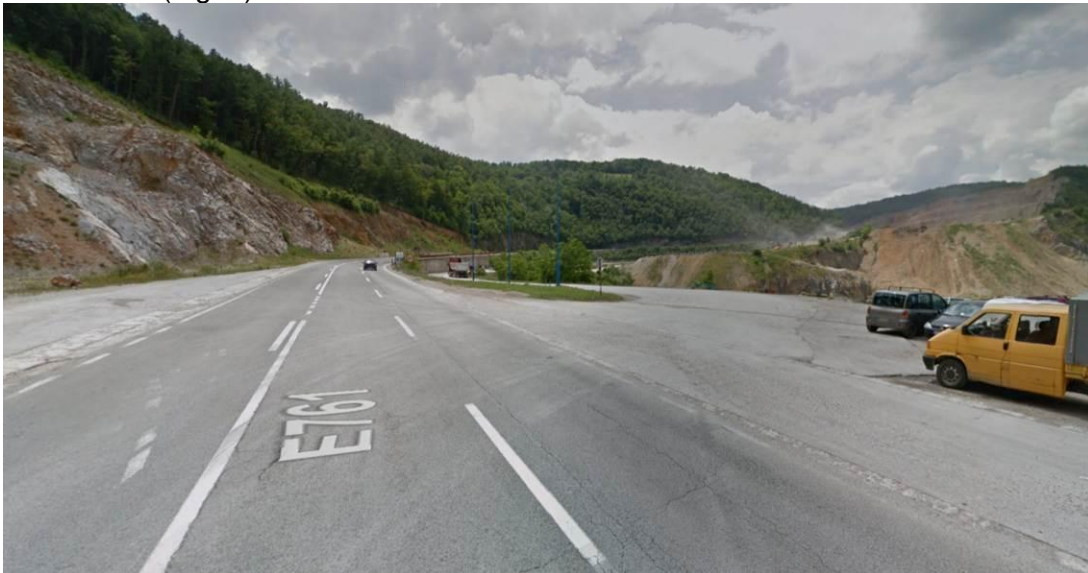
Figure 4. Connecting the access road to the quarry the relevant section km 148 + 760.00
