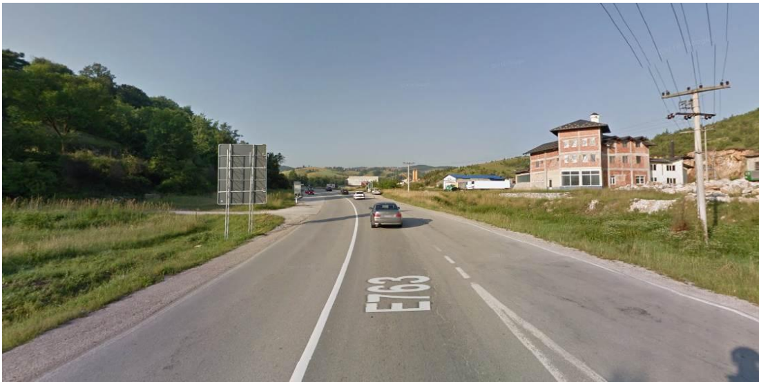
Figure 2. The end of the Section, end of the connecting ramp of the loop Susica
