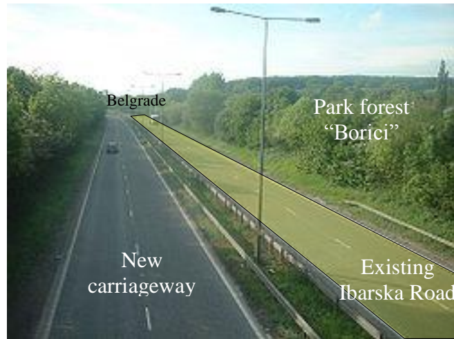
Example of Dual carriageway concept of future Ibarska road within the Park-Forest zone
